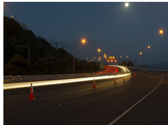
NGAURANGA TO AOTEA QUAY SMART MOTORWAY
