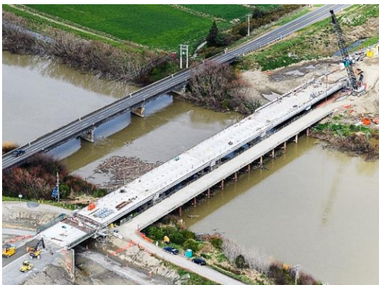
WHIROKINO TRESTLE AND MANAWATU RIVER BRIDGE
